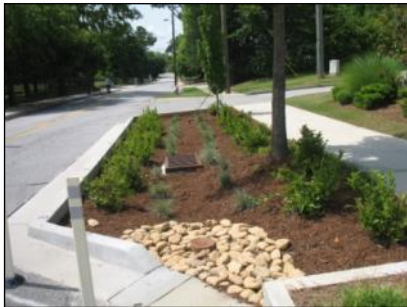
Bioretention - Whitehall Terrace ROW
