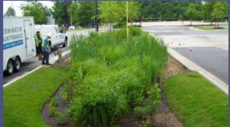
Micro-bioretentation in a parking lot
