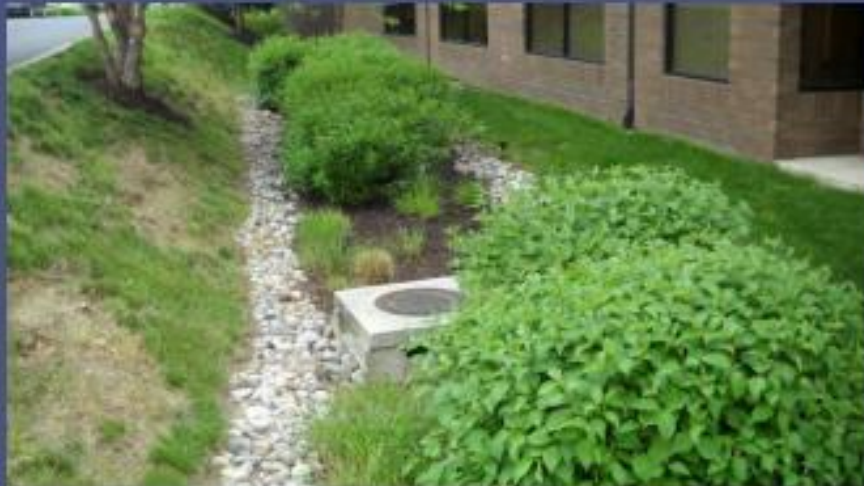
Micro-bioretentation adjacent to a building
