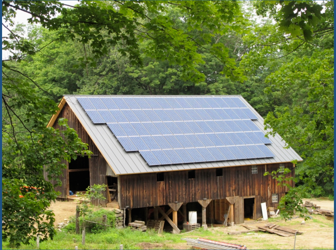
Dummerston, Vermont barn with 18 kW “group-net-metered” PV system - photo: Alex Wilson
