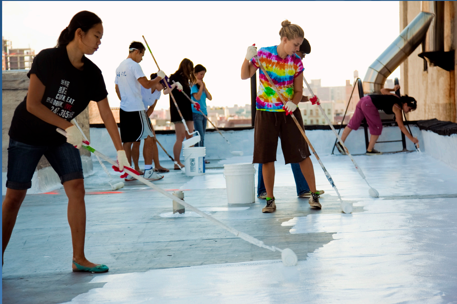
Volunteers painting a dark roof with reflective white elastomeric paint on the Bowery Mission in New York City, 2010 – photo: David Epstein
