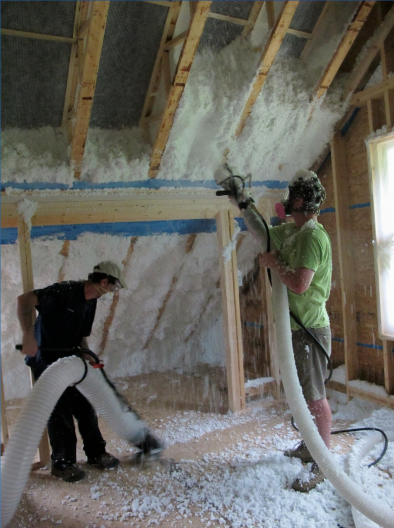
Johns Manville Spider spray fiberglass insulation – photos: A Wilson
