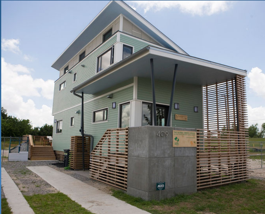
Post-Katrina home in New Orleans' Lower 9th Ward that is raised 4 feet. Global Green project & photo
