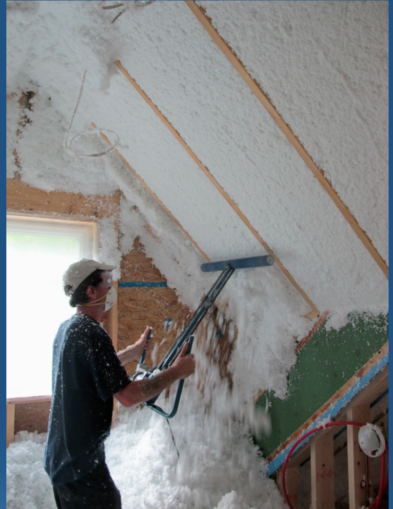
Johns Manville Spider spray fiberglass insulation – photos: A Wilson
