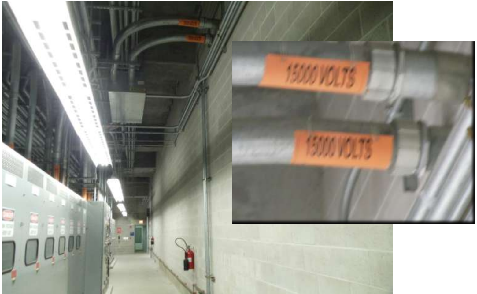
Vent Building 4— Detail of 15KV Electrical Conduit
