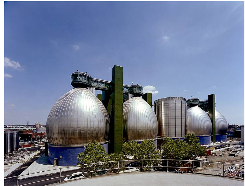
Existing anaerobic digesters at Newtown Creek waste water treatment plant in Brooklyn, NY
