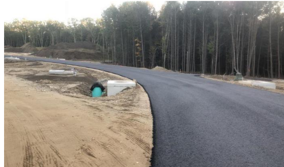
BIOSWALE WITH PRETX CATCHBASINS
