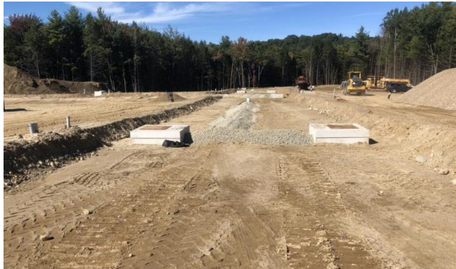
INFILTRATION TRENCH WITH PRETX CATCHBASINS
